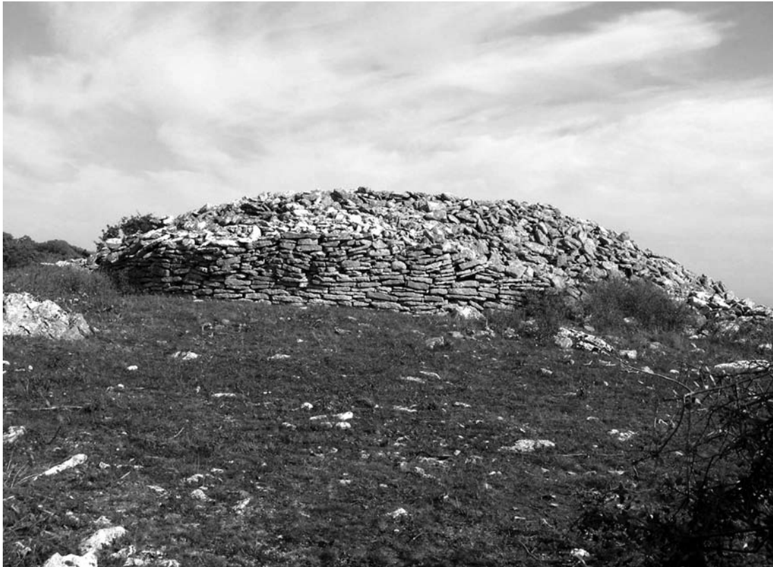
Figure 3. Lauphargi, the undamaged west wall (photo by R. Larje).
